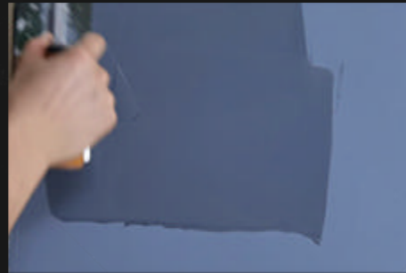
④ Apply 1-2 times in batch on the wall surface, and at least 4-6 hours interval for each time at normal room temperature
